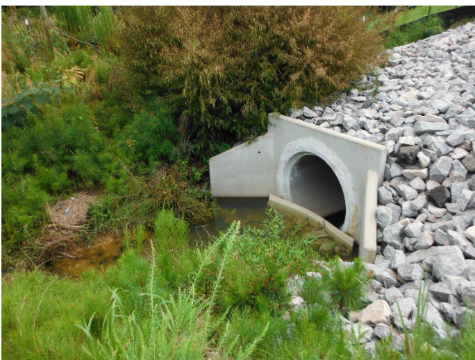
Lower reach pipe inlet prior to add. remediation July 9, 2025
