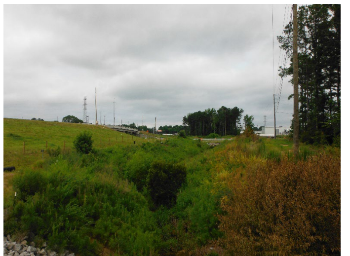
Overview of lower reach looking upstream from pipe inlet
