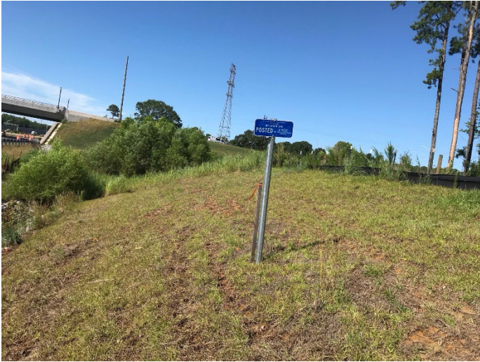
Mowed buffer along I-95 S back slope
